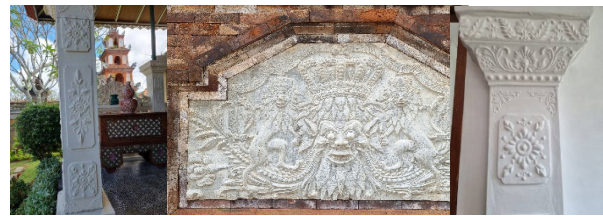
Figure 7. European-style ornaments with concrete moulding technique on the Gedong Maskerdam building (Source: Author's Documentation, 2024)
