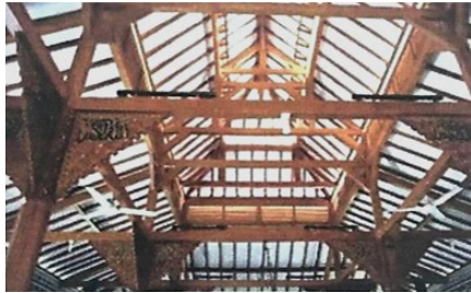
Picture 19. The ceiling is placed behind the roof structure (Source : Author, 2020)
